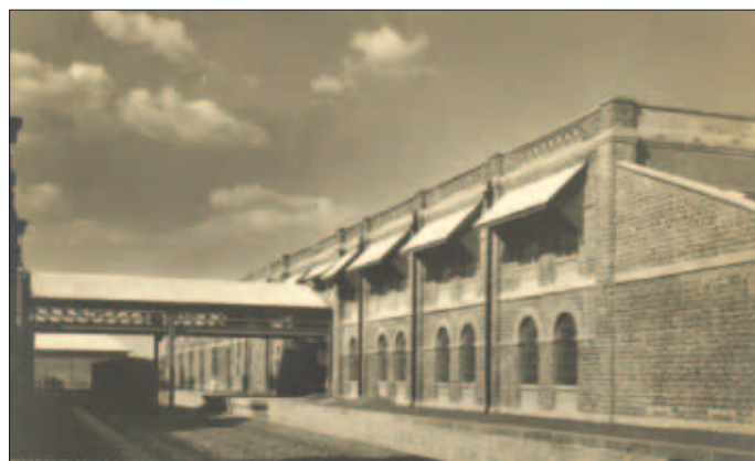
The Currency Note Press is just behind Security Printing India and separated from it by the railway line. The Central Stamp Store is also in this building.
